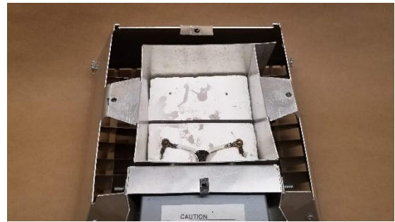
2. Disconnect and remove old element
