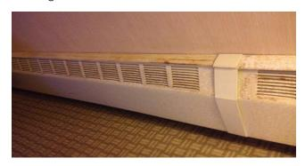
Hot air spreads out, becoming less dense and rising in the air. This creates a vacuum, pulling cool air towards the baseboard heater and starting the process over again. A natural convection process takes place as cold air enters the bottom of the element, is heated and then lifted as it comes in contact with the hot element and released back into the room. While baseboard heating is inexpensive to install, it has several drawbacks.
